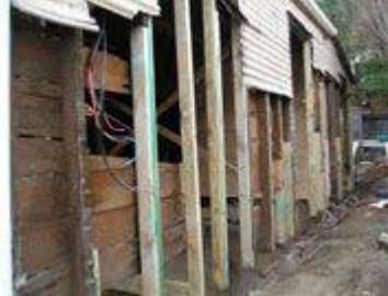
Relocation Preparation - 5 July 2005
