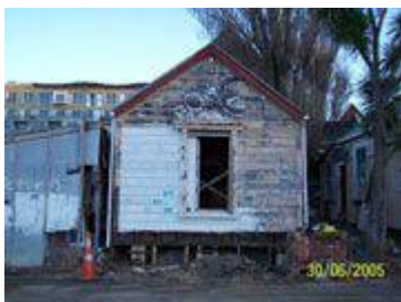
Relocation Preparation - 30 June 2005
