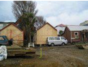
Relocation Preparation - 8 July 2005
