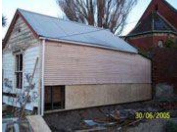
Relocation Preparation - 30 June 2005
