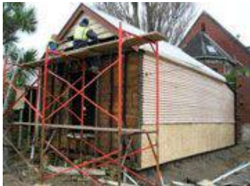
Relocation Preparation - 5 July 2005
